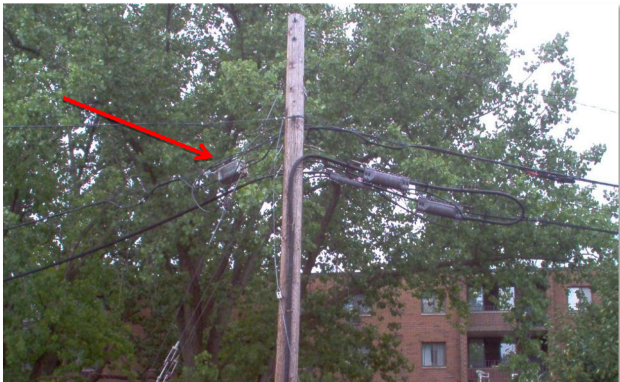
Figure 21: Utility Pole with Cable Amplifier
