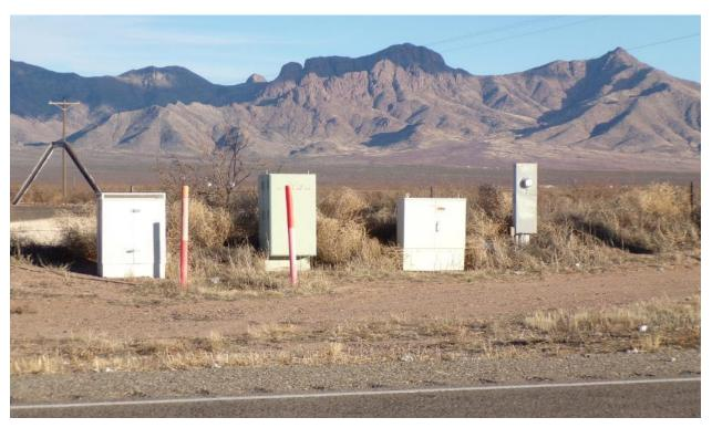
Figure 17: Deming Area – Transition From Fiber to Copper for Phone and/or DSL
